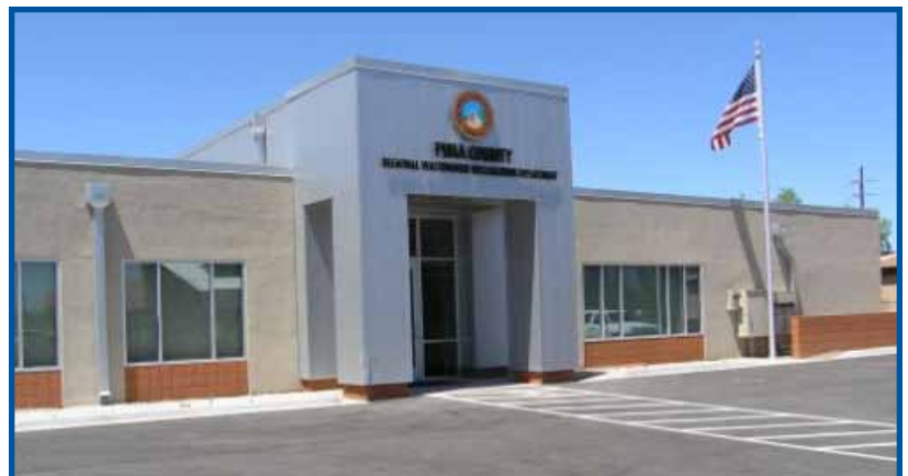
New Conveyance System Administrative Office
