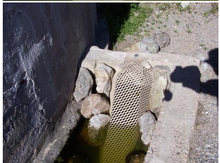
Photos 1 and 2: Wildlife escape ramps installed in A7 Ranch livestock drinkers. Ramps are designed to enable small animals, including bats, to escape the livestock waters.
