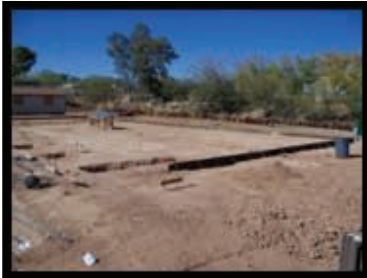
Construction Site for New Community Building
