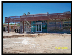
Catalina Building 75% Complete
