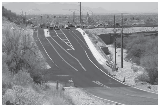
Sunrise Drive and Craycroft Road Intersection
