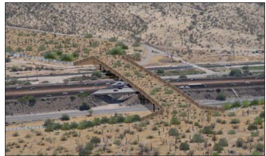
Artist's rendering of wildlife overpass. Photo by Coalition for Sonoran Desert Protection.
